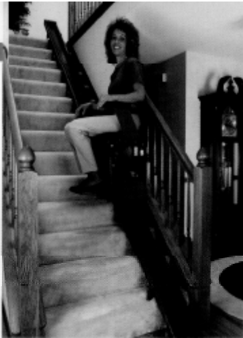
The stairway chair lift is an alternative to the vertical platform lift for clients who can make transfers.
