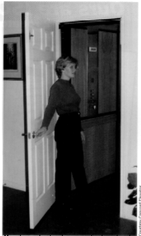
Many home elevators have an outer door at each stop that matches the design of the user's home.
